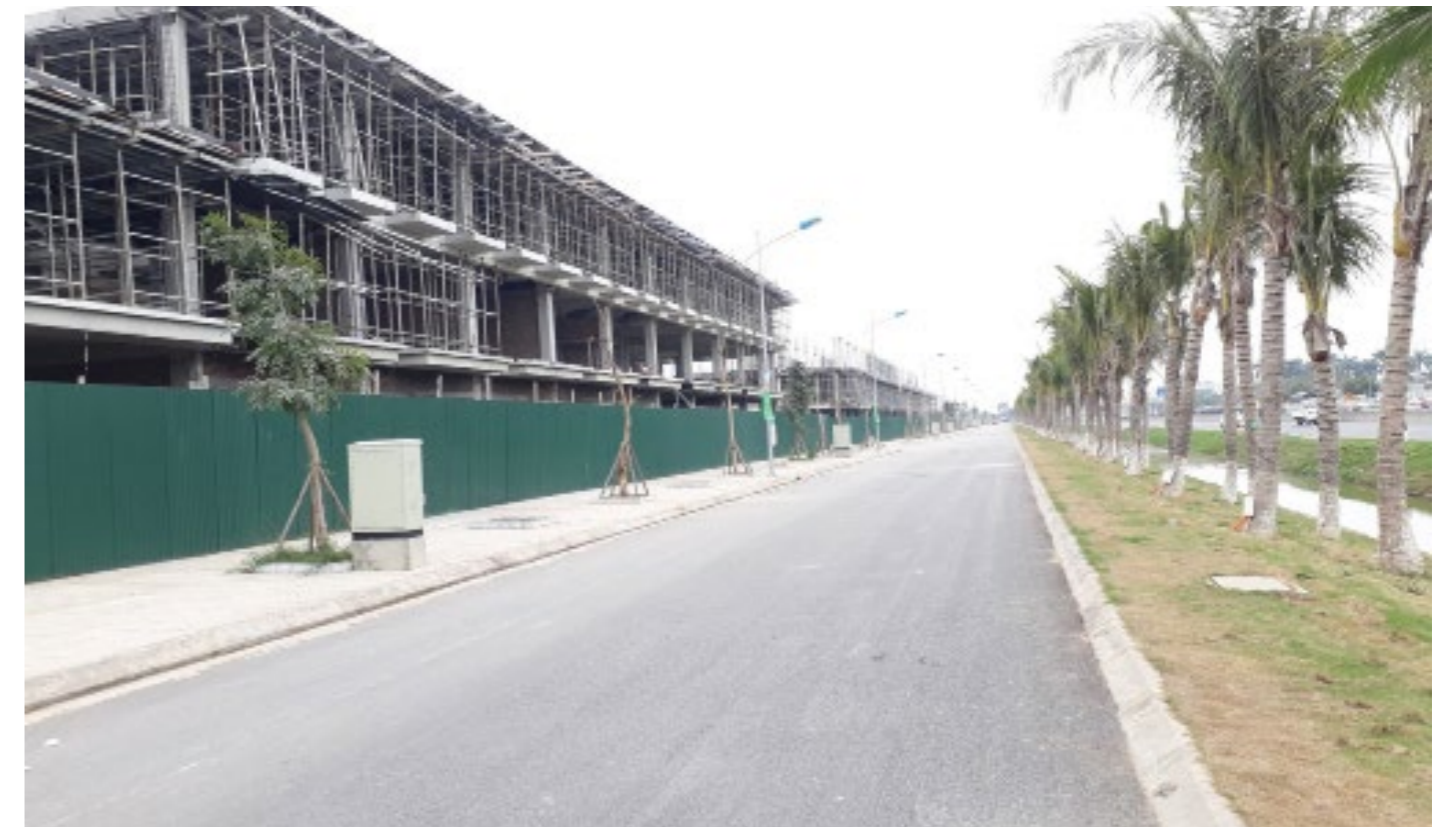
Trang Due Urban Area is deploying infrastructure and constructing commercial townhouses
